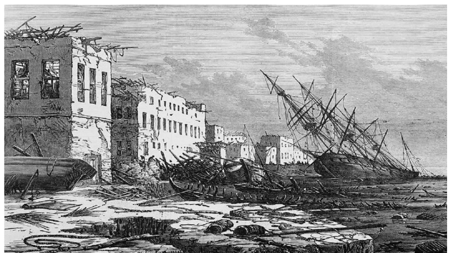
Figure 2. Historical artwork of the damage caused in Zanzibar harbour by the cyclone of 15 April 1872 (Science Photo Library, 2020). The accompanying caption from the Science Photo Library (2020) describes the following; 'Zanzibar is an island in the Indian Ocean, off the coast of present-day Tanzania. All the ships in the harbour, with the exception of a steamer that escaped to sea, were sunk or wrecked on the shore with great loss of life. The navy of the Sultan of Zanzibar was also wrecked, affecting his hold over the Arab seaports on the coast.'
