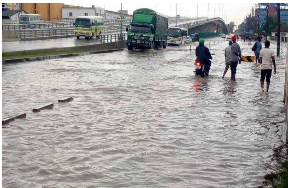
Figure 13: Impacts of heavy rainfall caused floods at Mandela road part of Mfugale flyover on 13 th October 2020 (Source: Habari Leo, 14 th October 2020).
